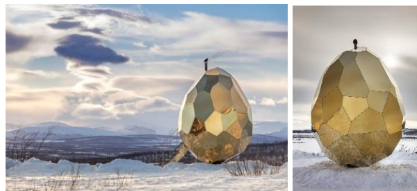
Figure 3-14. Solar Egg as an example of intentional aesthetic choice with futuristic solar power cladding. Image courtesy of ArchDaily. 145
